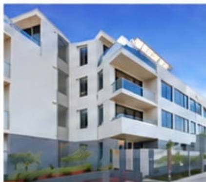
OCEANVALE 17 BUILDINGS (MERITON)
